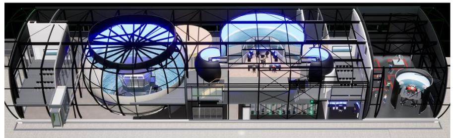
The Large Motion Simulator (on the left) in the SOSc with a moving bridge of 4 x 5 m on a hexapod and the Full Mission Bridge Simulator (in the middle).
